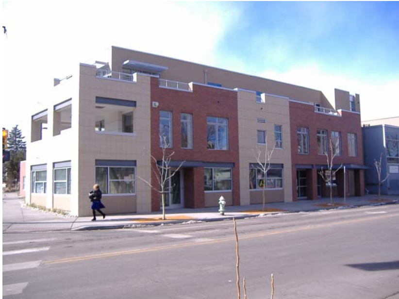
Easterly side- Looking northwesterly
